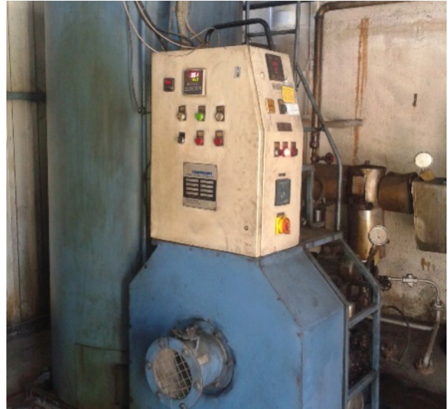
Biodiesel based boiler at Nashik
