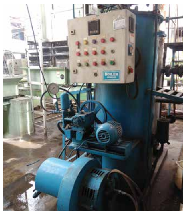
Biodiesel based boiler at our Nashik facility
